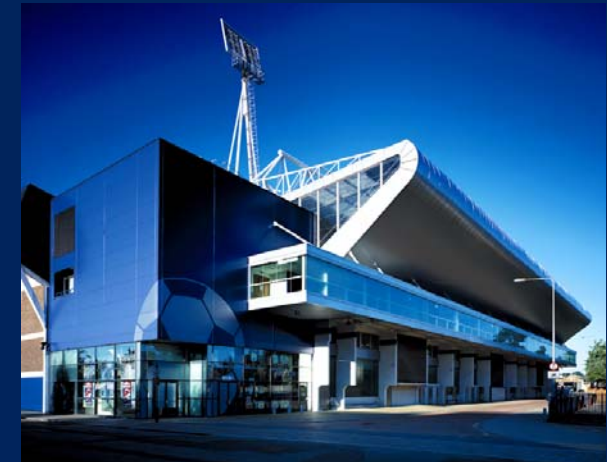
North Stand – Ipswich Town FC Jackson Construction £10m
